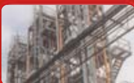
Chemical and Petrochemical Industries
